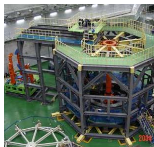
Completed Jig System (2004. 03)
