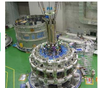
Install. of Central Solenoid (2006. 10)
