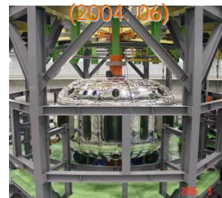
Re-construction of the Jig (2005. 03)
