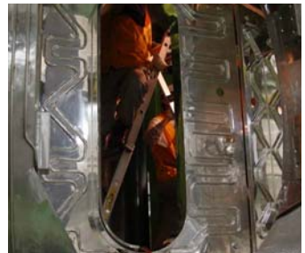
Install. of the VVTS Last Sector (2006. 06)
