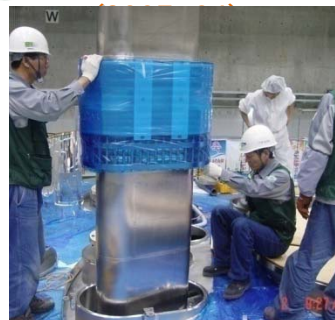
Assembly of VV Vertical Ports (2007. 05)
