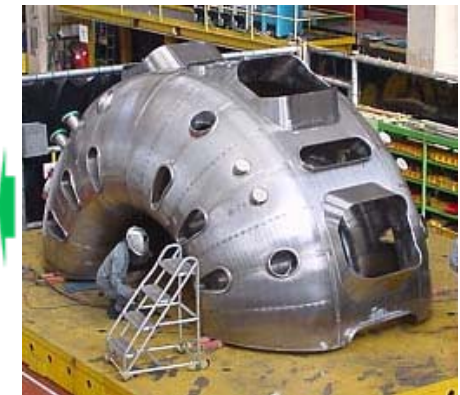
Welding of Sector 1
