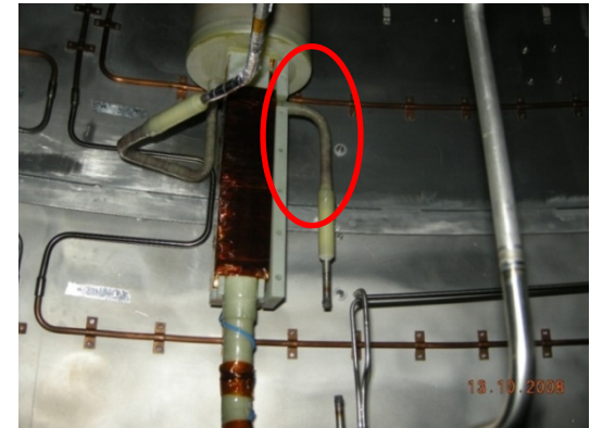
PF3,4,5U Lap joint case remove
