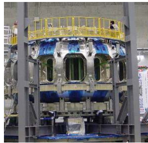
Install. of the PF6L & PF7L
