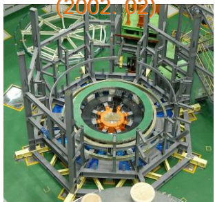
Pre-install. of PF6L & PF7L (2004. 07)
