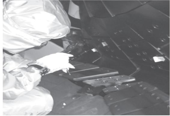
Fig. 7 Setup of divertor plates in vacuum vessel
