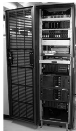
Fig.1. DS20E Tru64/VMS data storage and analysis system
