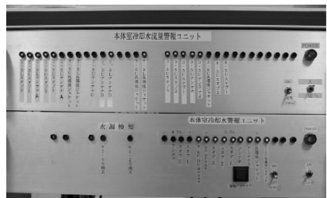
Fig.13 Stand-alone condition display system for the cooling water flow.
