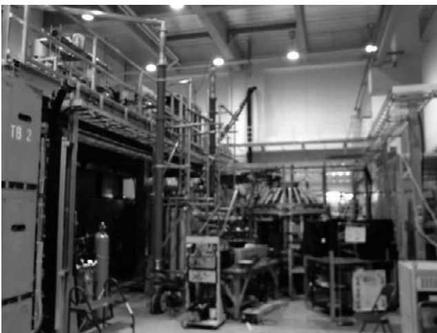
Fig. 1. Photograph showing the coaxial transmission lines to deliver RF power from 200 MHz transmitters to the two-strap loop antenna installed inside TST-2.
