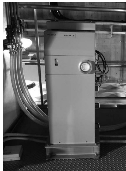
Fig. 16. Snap shot of the room gas monitor on the LHD experimental floor.
