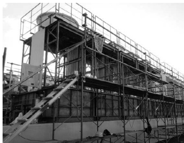
Fig. 11. Cooling Tower under construction.
