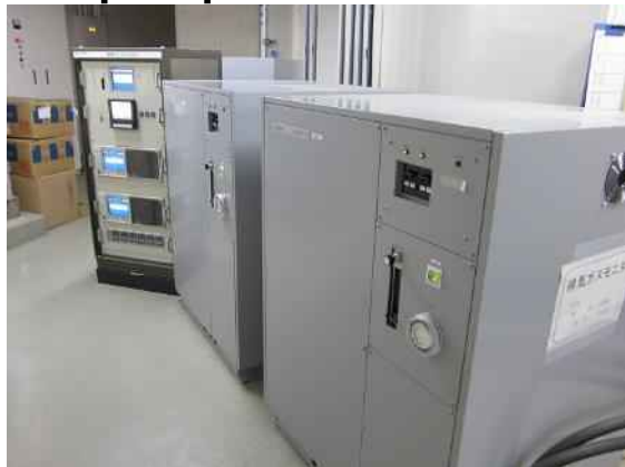
Stack gas monitors
