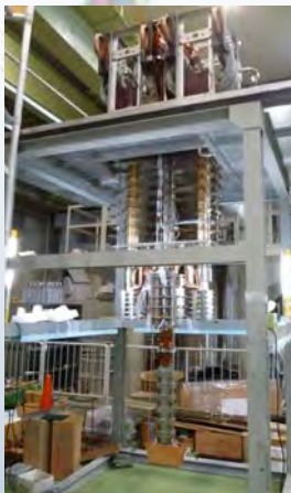
Performance test of the ITER-TF connection part in NIFS
