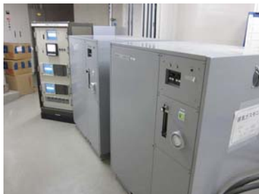
Stack gas monitors
