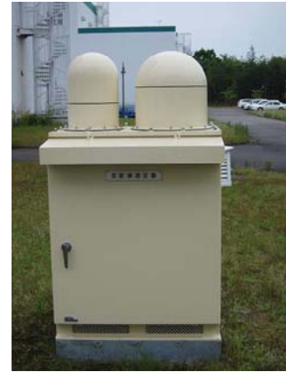
Monitoring post of RMSAFE
