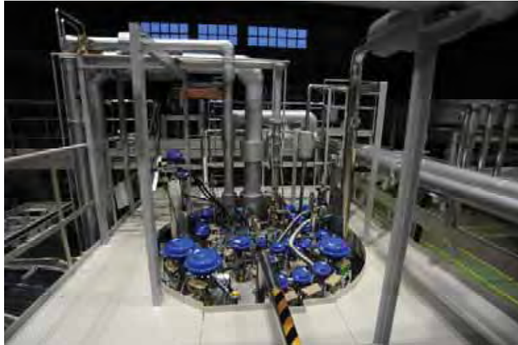
Figure 3.3.2.1-4 Photo of the refrigerator/liquefier.
