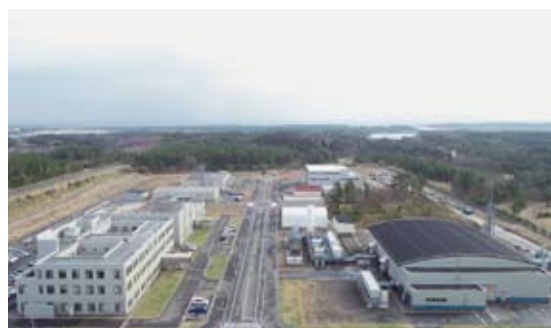
A panoramic view of QST Rokkasho Fusion Institute in Dec.2020 where the NIFS Rokkasho Research Center is located.
