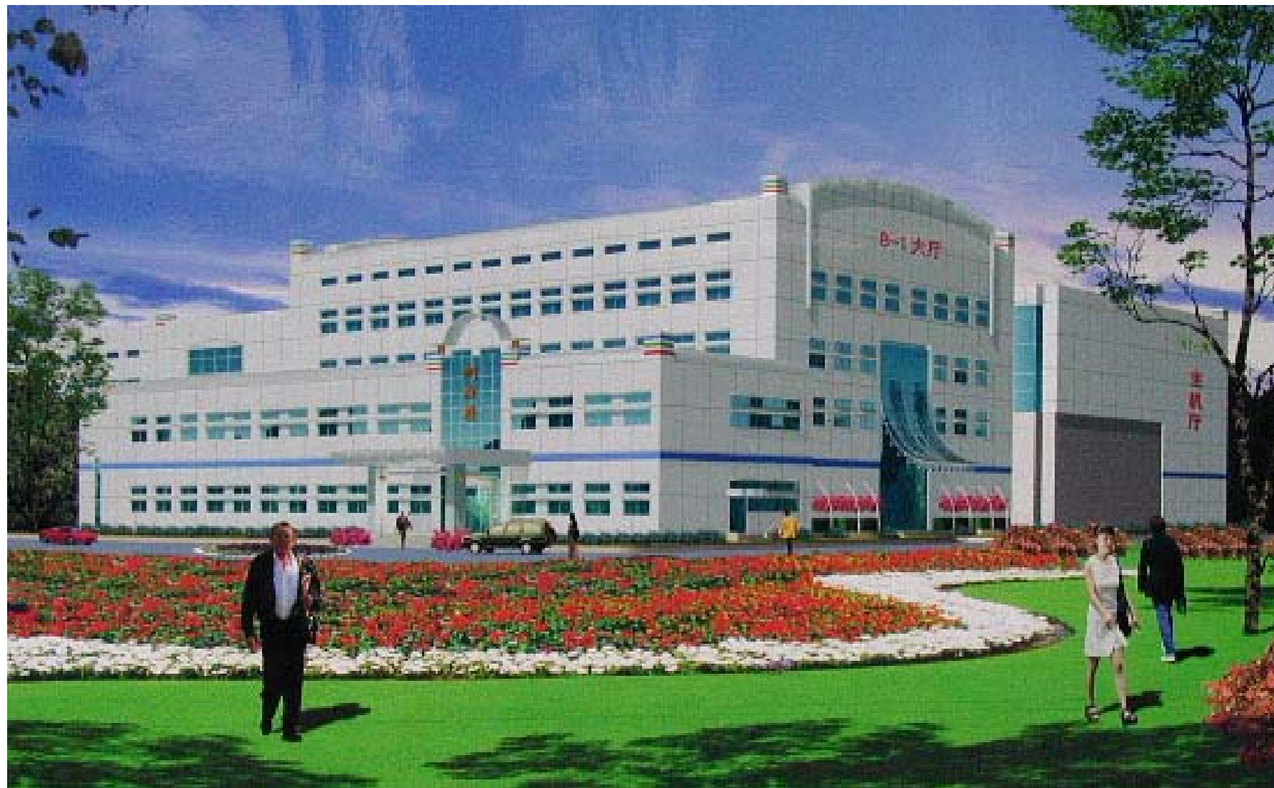
The building for HT-7U (will be completed around May 2002)
