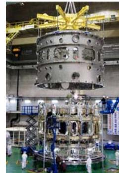
Fig.2 Assembly of the cryostat cylinder
