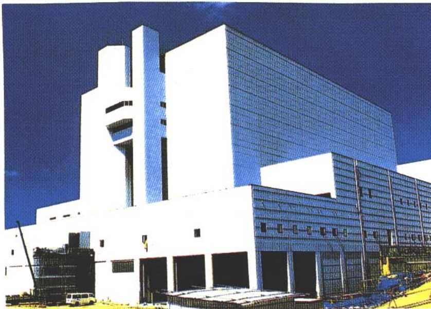
Fig.15 Photograph of LHD Experimental Building.
