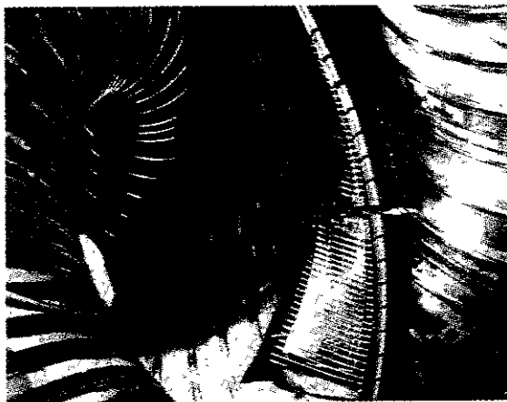
Fig.1 Photograph of ICRF loop antennas in LHD vacuum chamber
