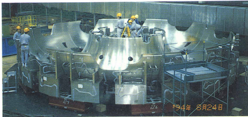
Figure 4 The completed lower supporting structure
