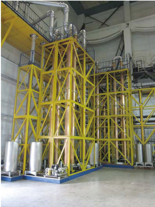
Fig.18 Impedance matching system with three Liquid stub tuners
