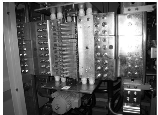
Fig. 27 The polarity switches for the power supply.
