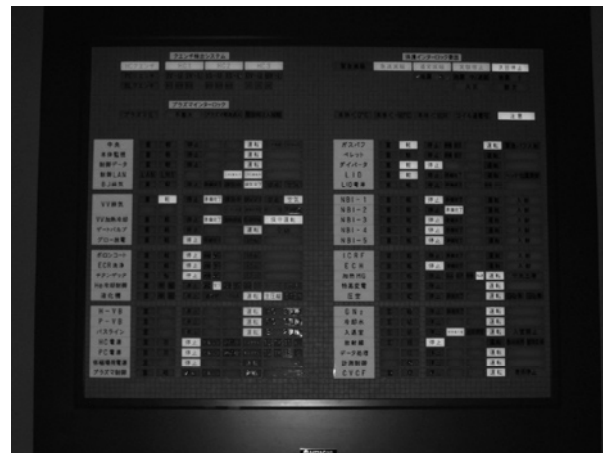
Fig. 27 Display of the central control system for LHD
