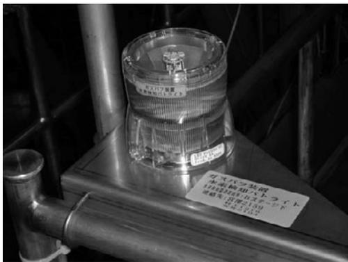
Fig. 13. Installed a revolving light for a H2 detector
