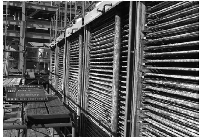
Fig. 14. Replacement of the Cooling tower
