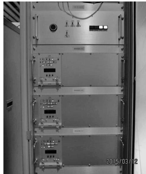
Fig. 2. Digital signal processing units and interface unit for the  $^{235}\text{U}$  fission chamber.
