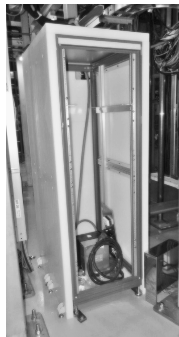
Fig. 10. Control panel was covered by white polyethylene block ( t = 50 mm).
