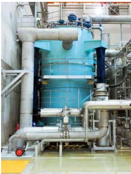
Fig. 2 Photograph of helium refrigerator/liquefier for the LHD.
