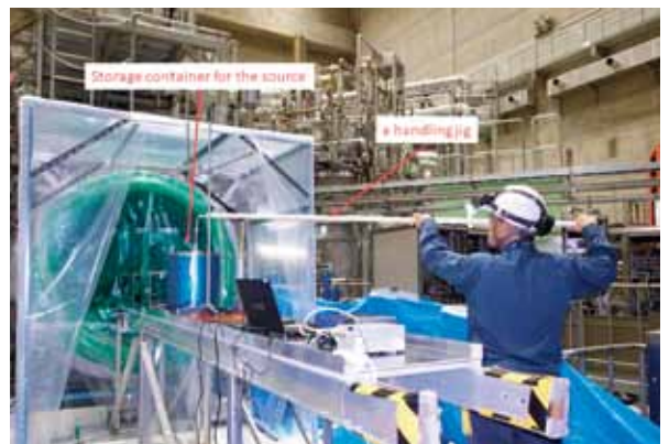
Fig. 8 Installation of the absolutely calibrated neutron source for in-situ calibration of NFM.
