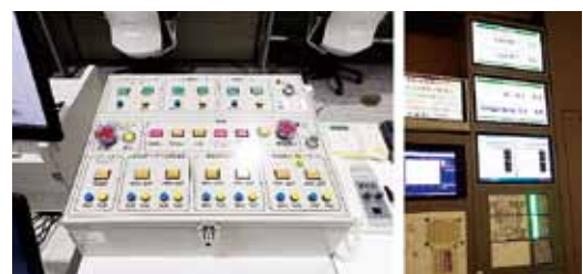
Fig. 11 The control console and the integrated monitoring display installed in the control room
