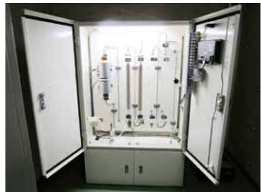
Fig. 10 The newly installed tritium sampler
