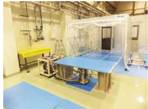
Fig. 8 Overview of the maintenance room
