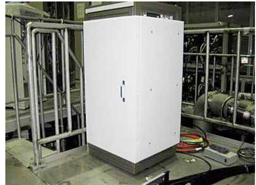
Fig. 9 19-inch system rack covered by polyethylene plates
