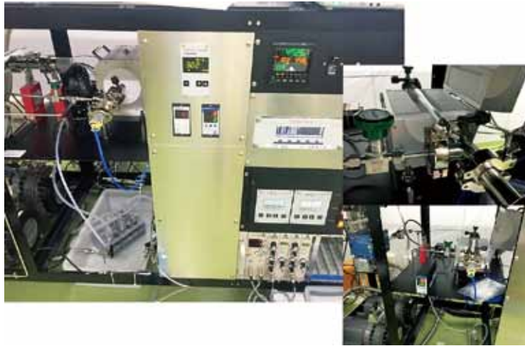
Fig. 14 The HI-TDS system installed in the LHD building at NIFS.
