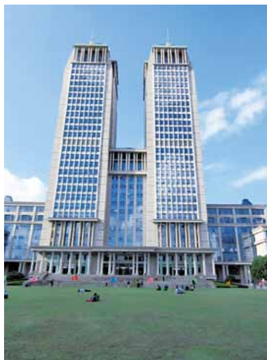
2017/Oct. Faculty building for cultural affairs in Fudan University in Shanghai, China. Shanghai-EBIT device is installed in Fudan University and collaborations are made on atomic physics with Tokyo-EBIT in University of Electro Communications, and on fusion research with ASIPP at Hefei, China and NIFS at Toki, Japan.
