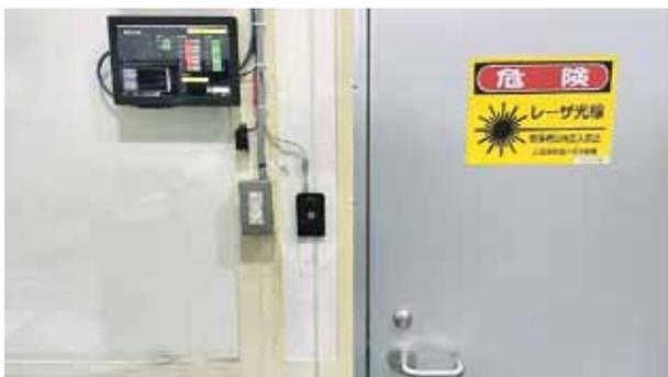
Fig. 16 Laser room interlock system in operational check
