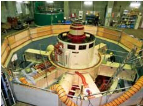
Fig. 10 Motor disassembly (A motor is on the stay. There is a generator under the stay)
