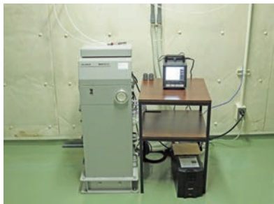
Fig. 16 3rd gas monitor in air conditioning room
