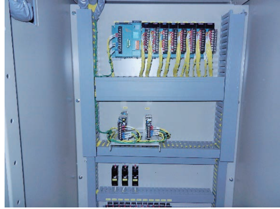
Fig. 11 The updated PLC of speed control panel
