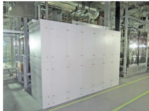
Fig. 13 Radiation shielding by high density borated polyethylene blocks
