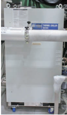
Fig. 14 Water cooled refrigeration type chiller for YAG Thomson scattering system
