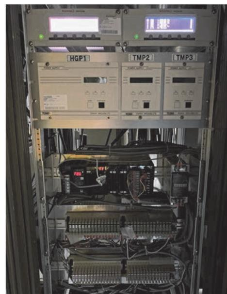
Fig. 20 PLC and controllers of the TESPEL#4.
