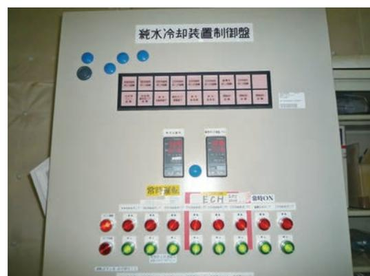
Fig. 7 Cooling water pump control panel on/off button (8 systems)
