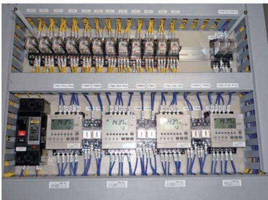
Fig. 6 Additional 2ch timers and relays (8 systems)
