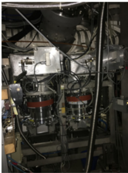
Fig. 6-4 Picture of vacuum pumping system for CHS
