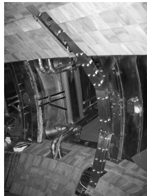
Fig.8 Dedicated ICRF antenna for wall conditionings in EAST
