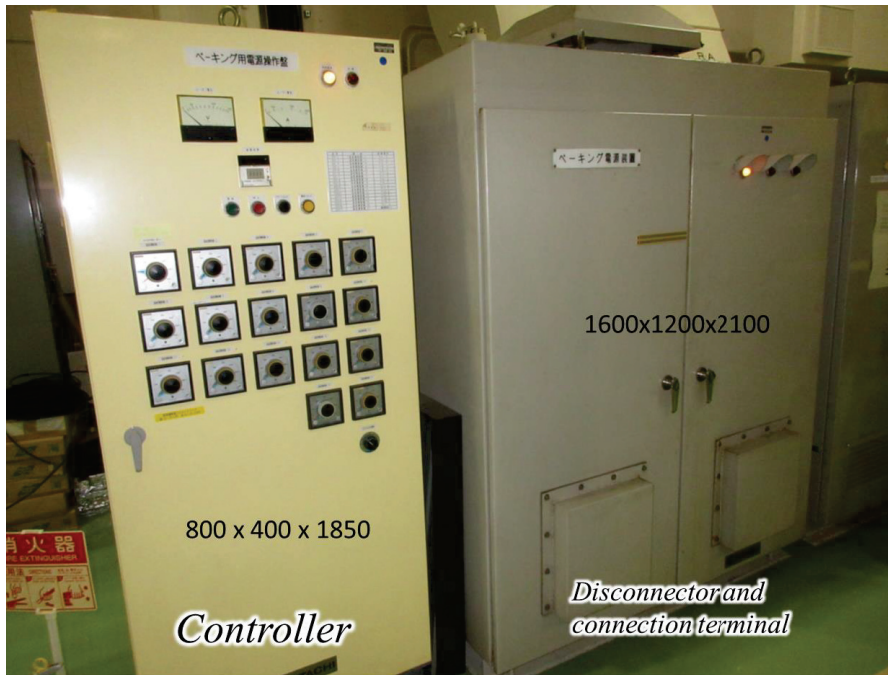
Fig. 3.6.1 Power supply for baking vacuum vessel.
