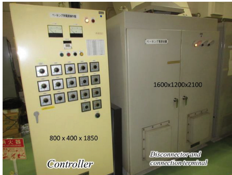
Fig 1.6-1 Power supply to bake the vacuum vessel for the CHS.
