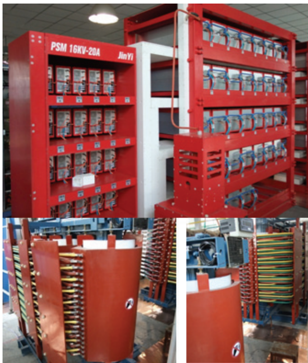
Fig. 3 PSM power supply for TH535 and TH525A tetrodes
