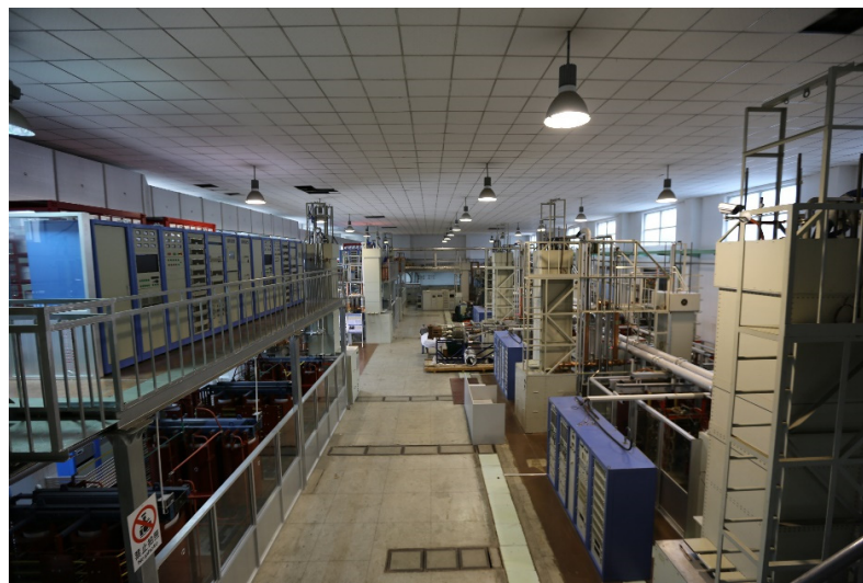
Figure 1 View of 12.0 ICRH system In EAST ICRF hall
