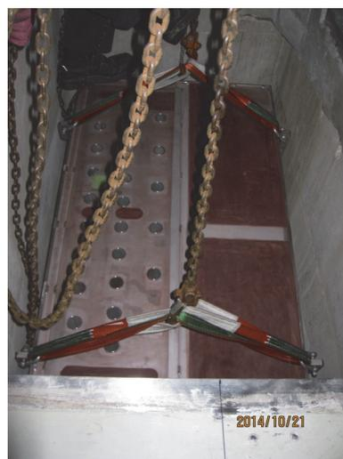
Fig. 6 Installation of the neutron collimator made of heavy concrete.
