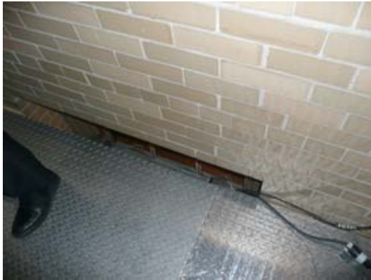
Fig. 25. Stage at the capacitor bank area.
