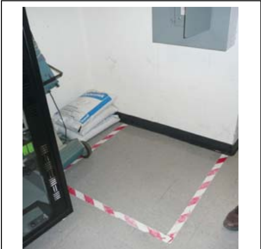
Fig. 20. Partitioning off the front area of the power supply board.
